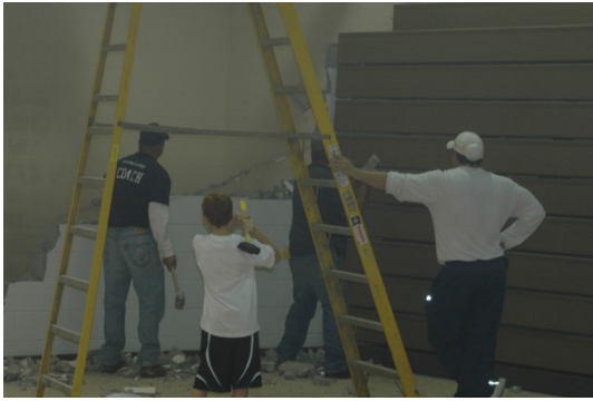
John Miller and Kurt Thelen demolish one of the storage closets while Daric Feldpausch supervises and Tony Hufnagel waits his turn.
